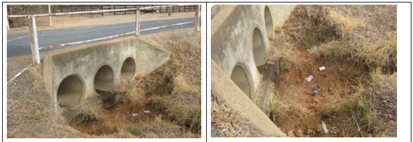
Figure 7-2: Existing Stormwater Outlet 1
