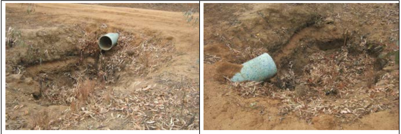
Figure 7-3: Existing Stormwater Outlet 2
