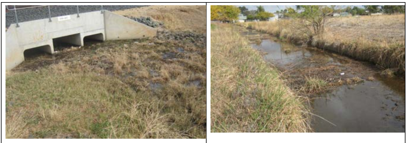
Figure 7-4: Existing Stormwater Reach 1
