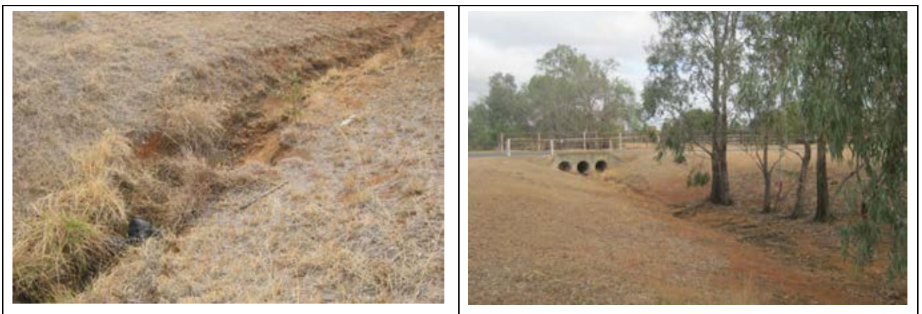
Figure 7-5: Existing Stormwater Reach 2
